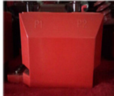
Resin current transformer
